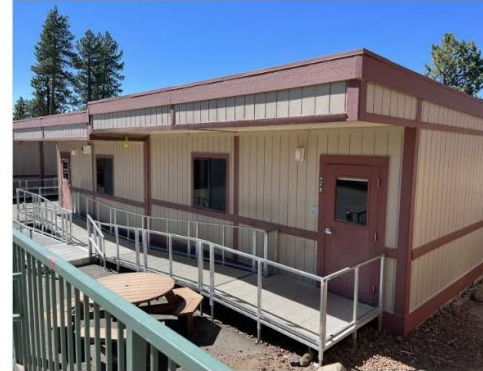
Replacement of portables with permanent structures
