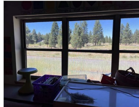
Snow removal access needed for windows
