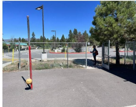
No shade structure over playground
