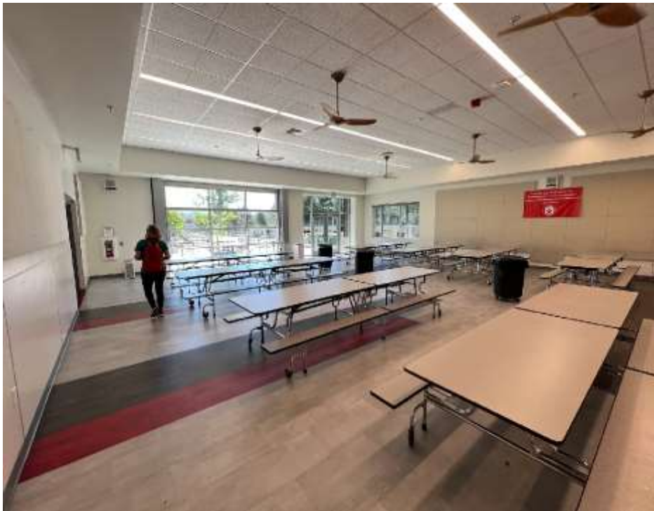
Undersized core facilities
