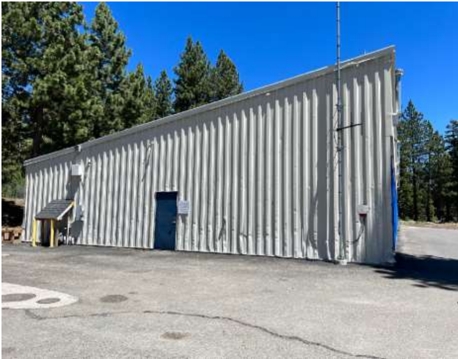
Exterior lighting and facade upgrades
