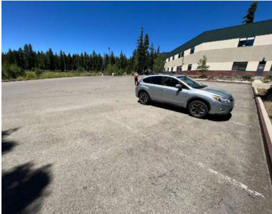
Parking lot asphalt upgrades
