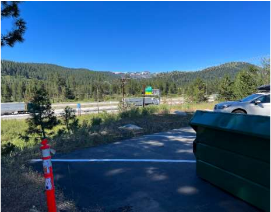
Parking additions and ADA upgrades
