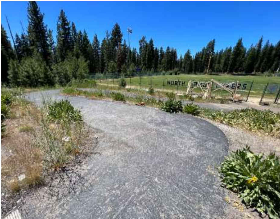
ADA path upgrades to the field
