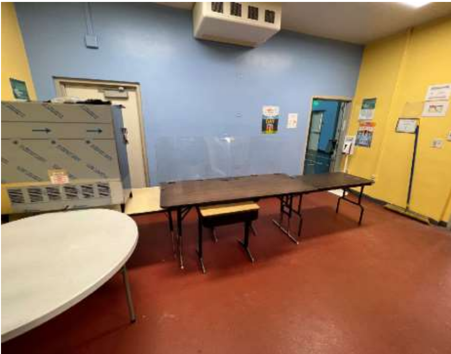
Kitchen expansion and modernization
