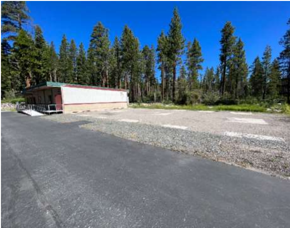
Pave existing gravel
