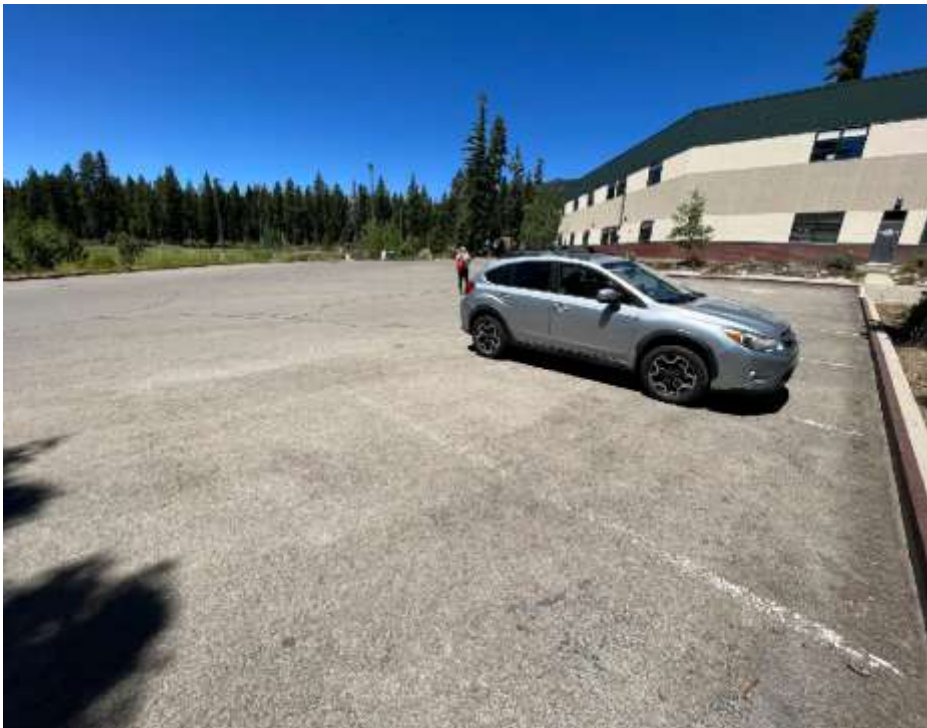
Parking lot asphalt upgrades
