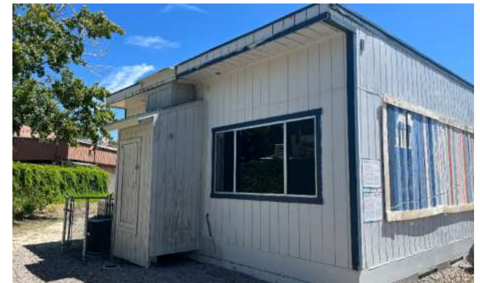
Replacement of portables with permanent facilities
