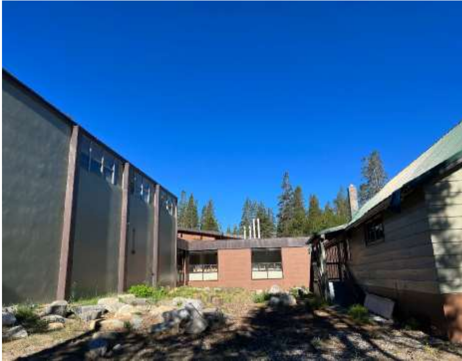
Roofing replacement and exterior renovation
