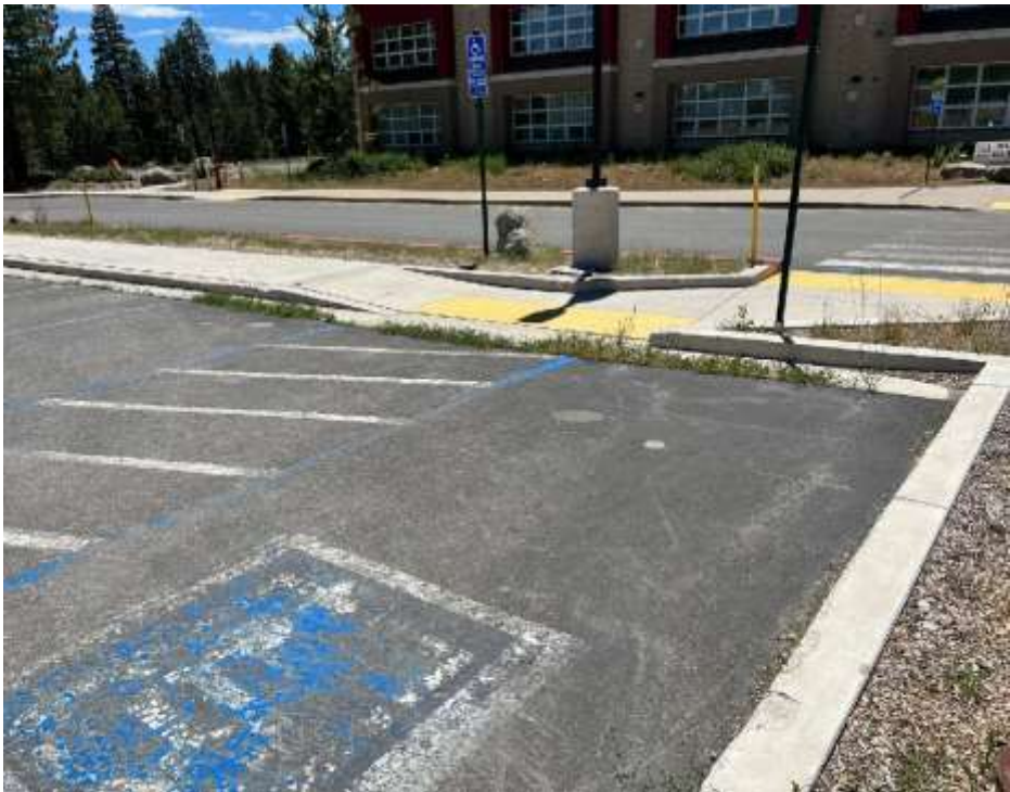
Asphalt in parkinglot and drop-off paving upgrades
