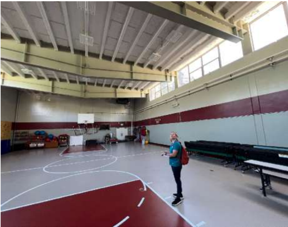
Aging core facilities
