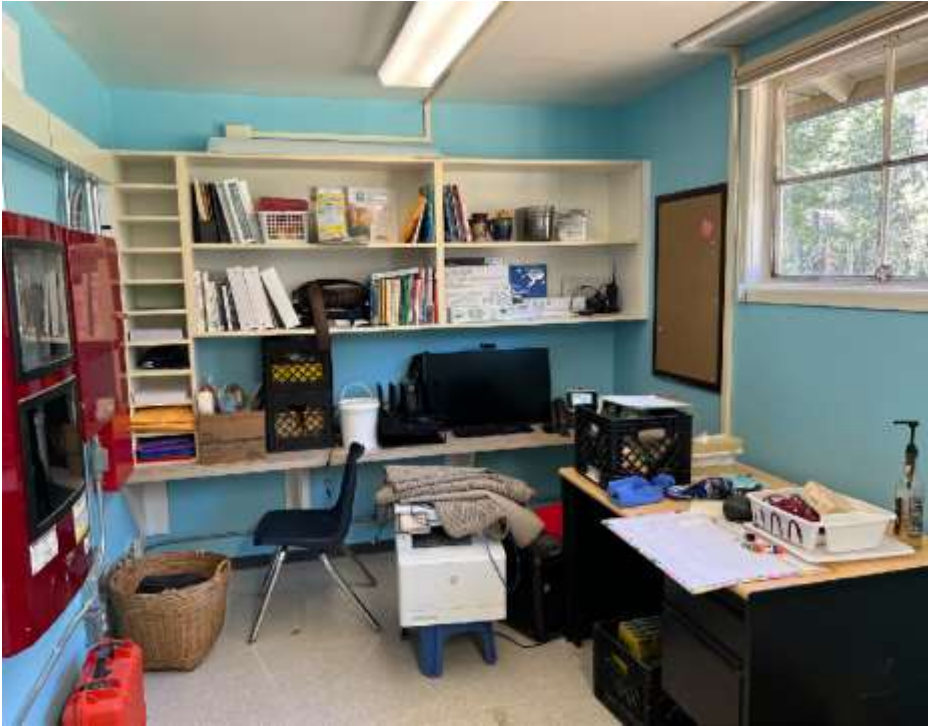
Office casework and interior finish upgrades
