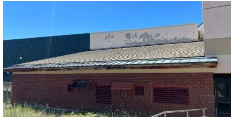
Refresh of some exterior finishes
