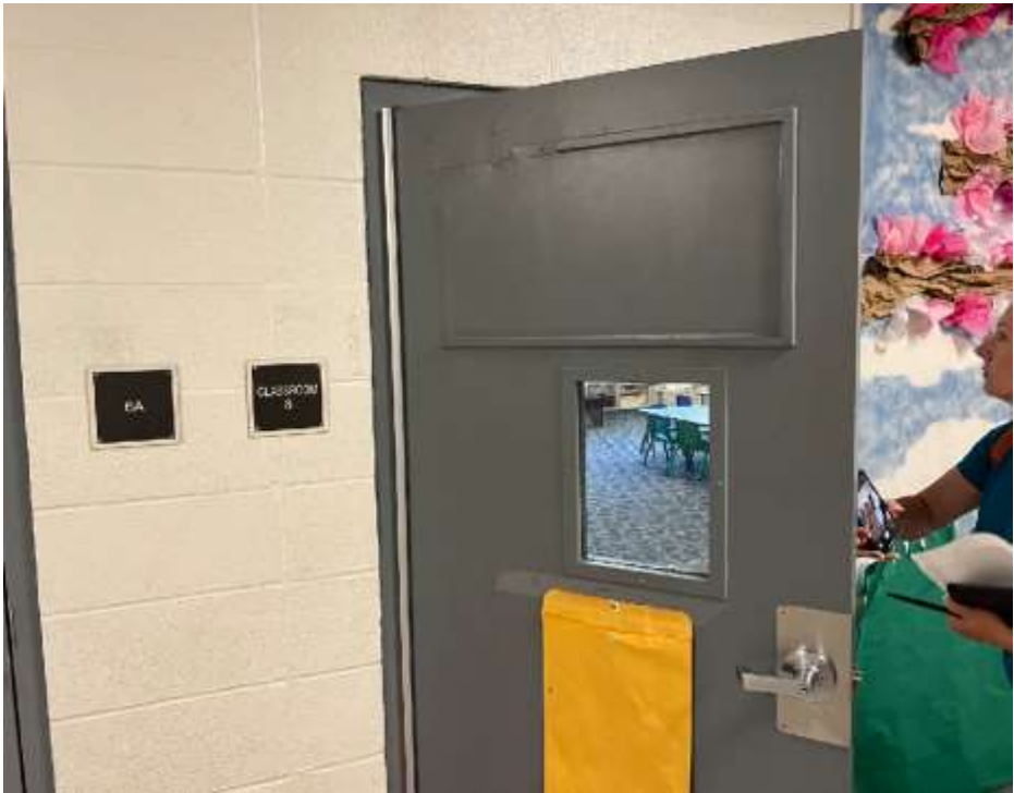
Classroom door and interior renovations
