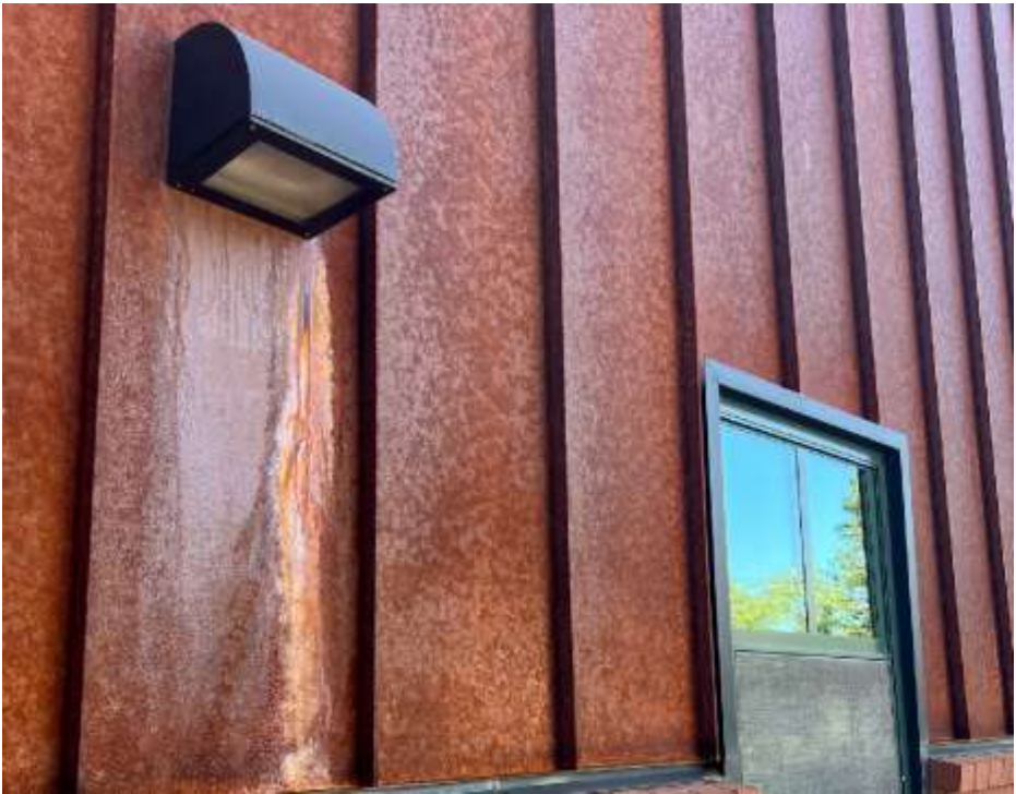
External metal replacement
