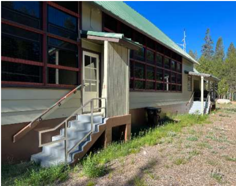
Emergency exit and site landscape upgrades
