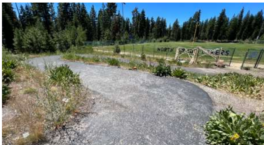
Accessibility needs at athletic facilities
