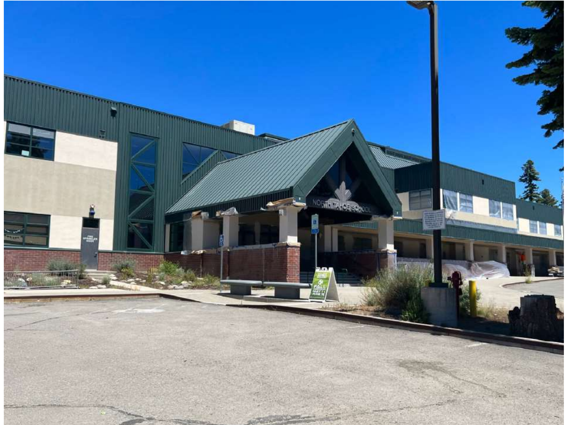
Entrance at North Tahoe Middle School
