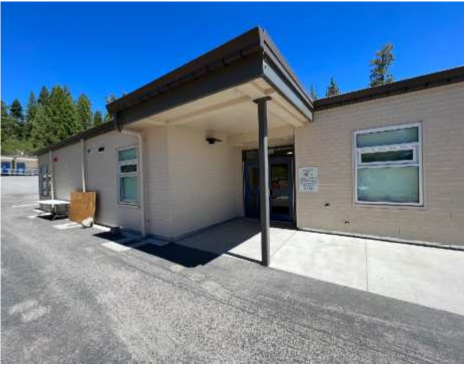
Roof, windows, and concrete upgrades
