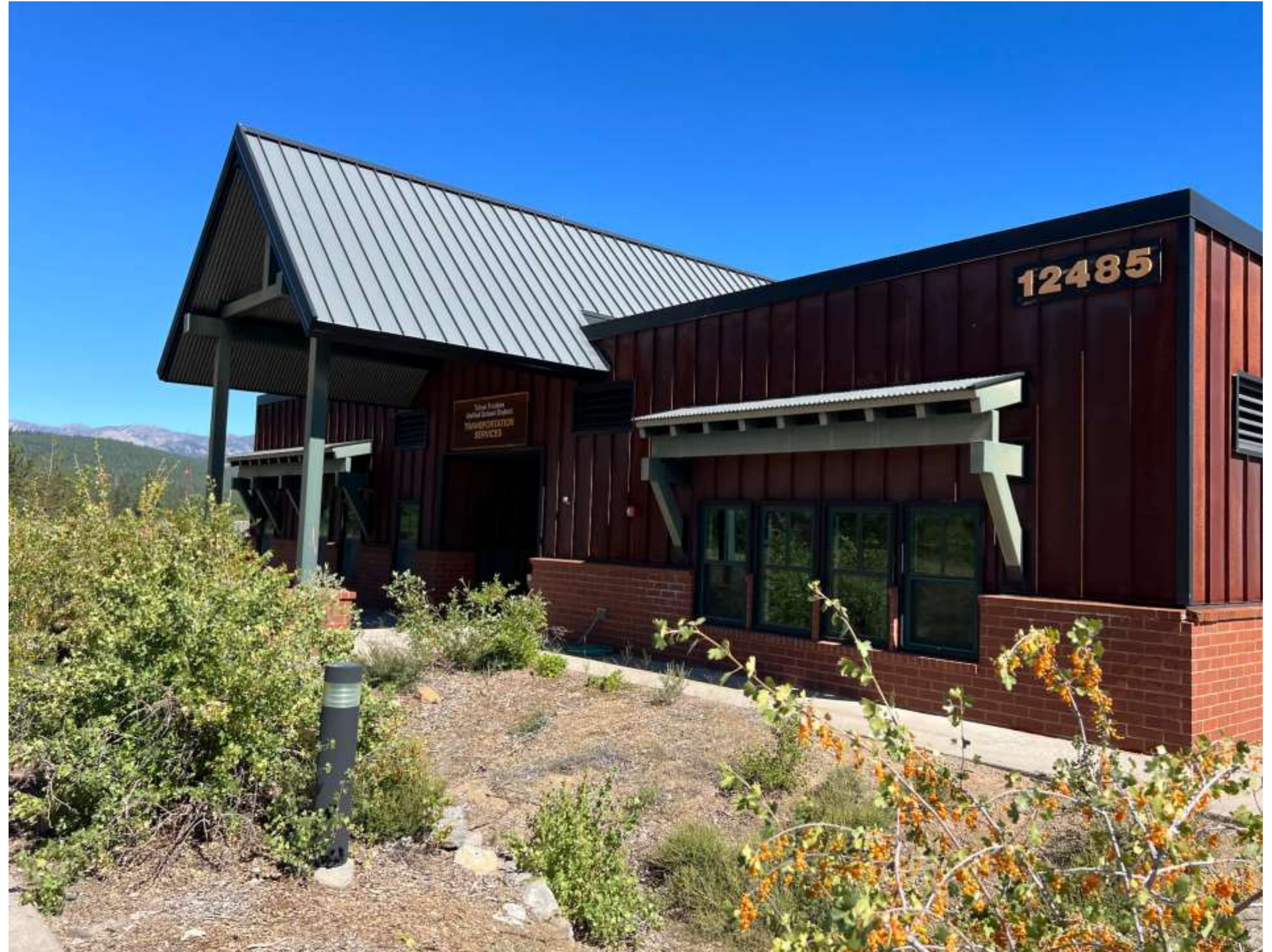
Entrance at District Transport and Maintenance Facility
