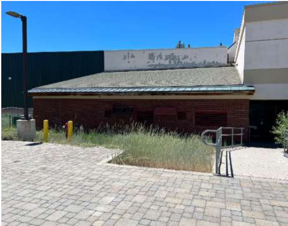
Exterior wall and paint upgrades
