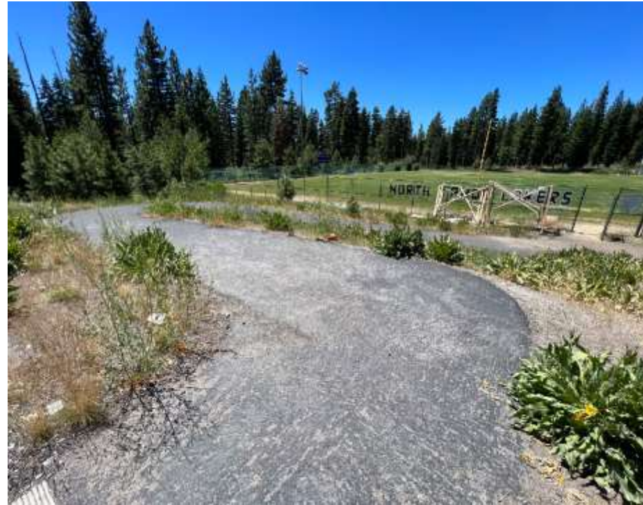
ADA path upgrades to the field
