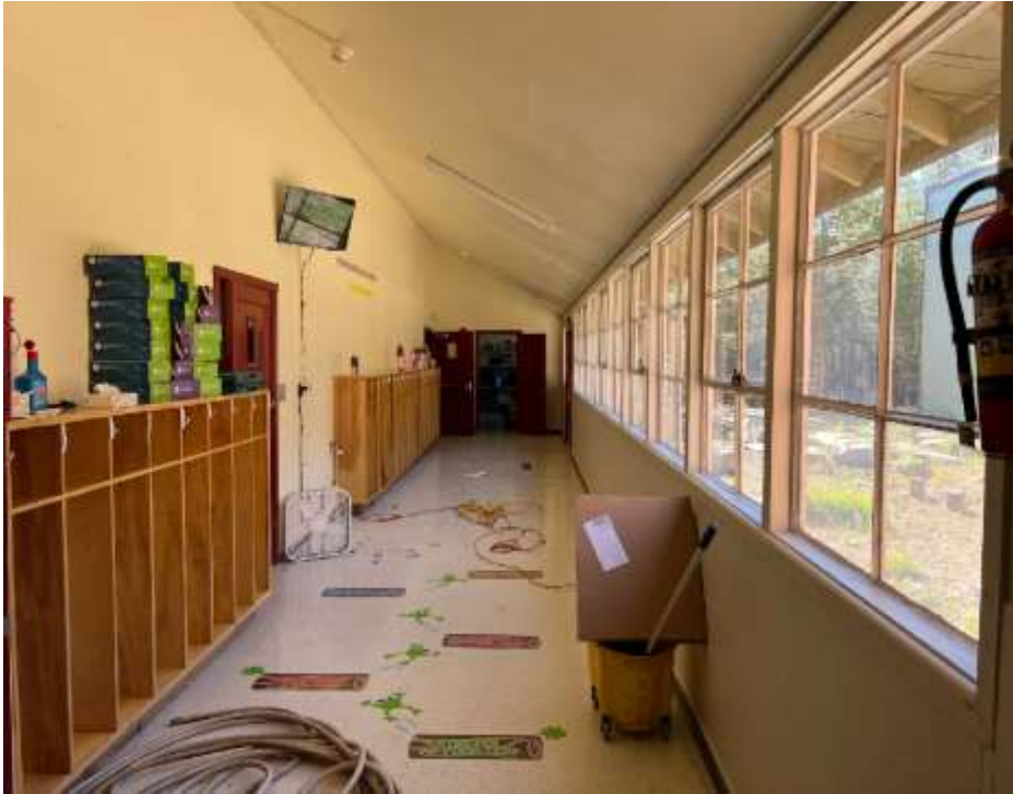
Interior finish upgrades and replacements
