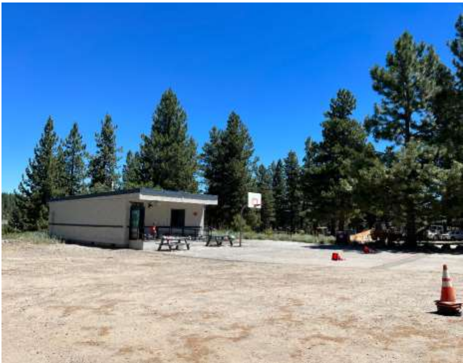
Landscape improvements and hardscape repavement
