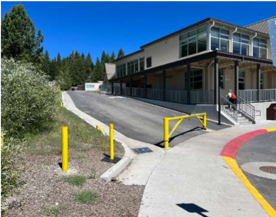
Single pane windows need replacing
