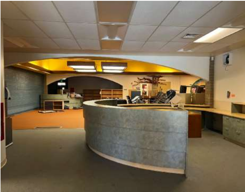
Modernize interior finishes and casework
