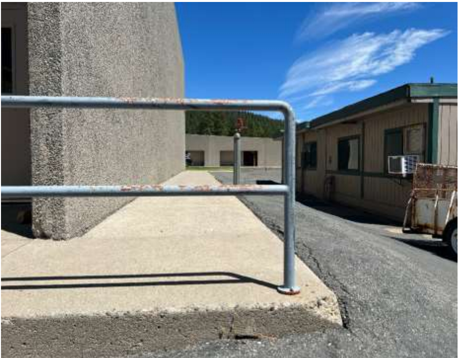
Curb, asphalt, and rusted handrail replacement
