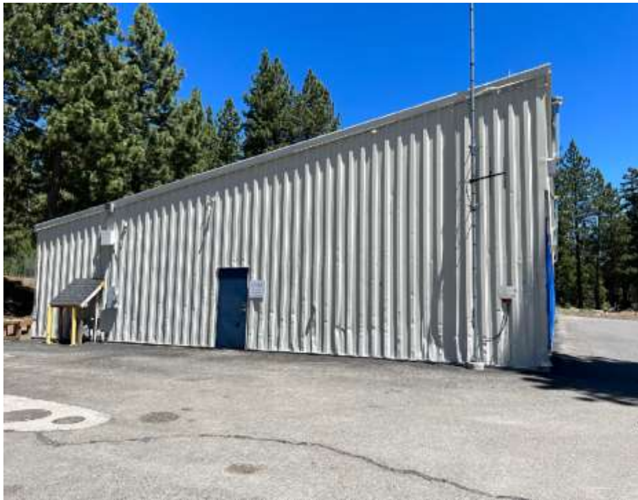
Exterior lighting and facade upgrades
