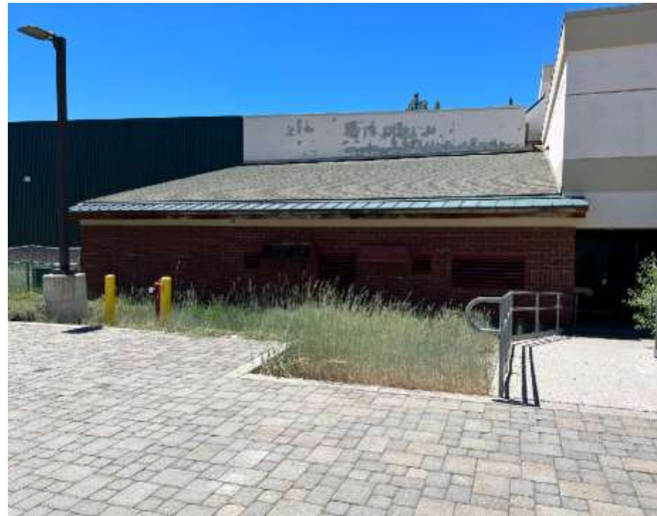
Exterior wall and paint replacement
