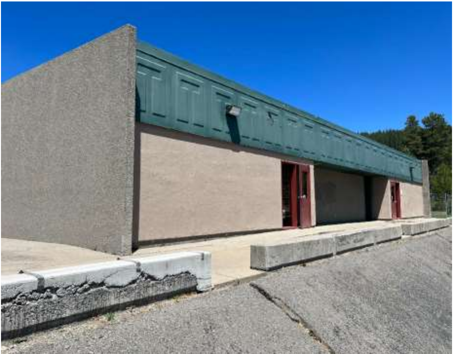
Hardscape and curb repaving
