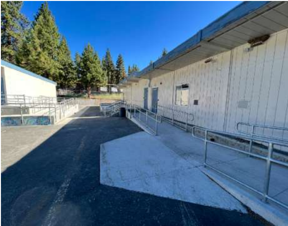
Portable building replacement
