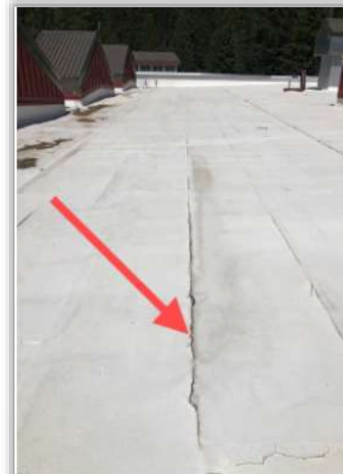
Long cracks have formed the the membrane
