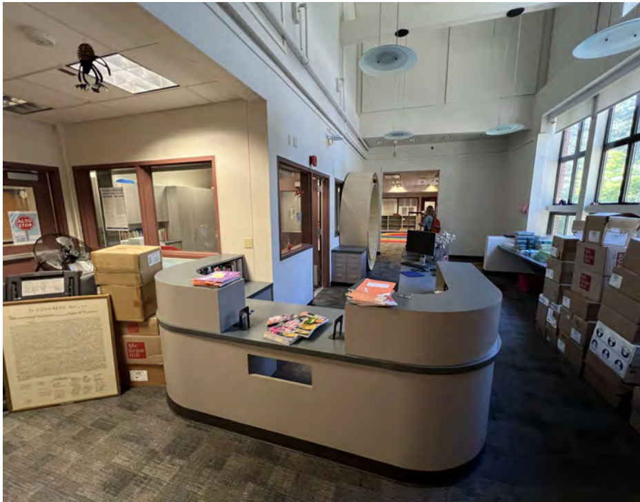
Library modernization and building infrastructure improvements
