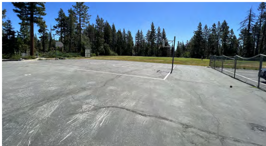
Repairs to paving from snow removal damage
