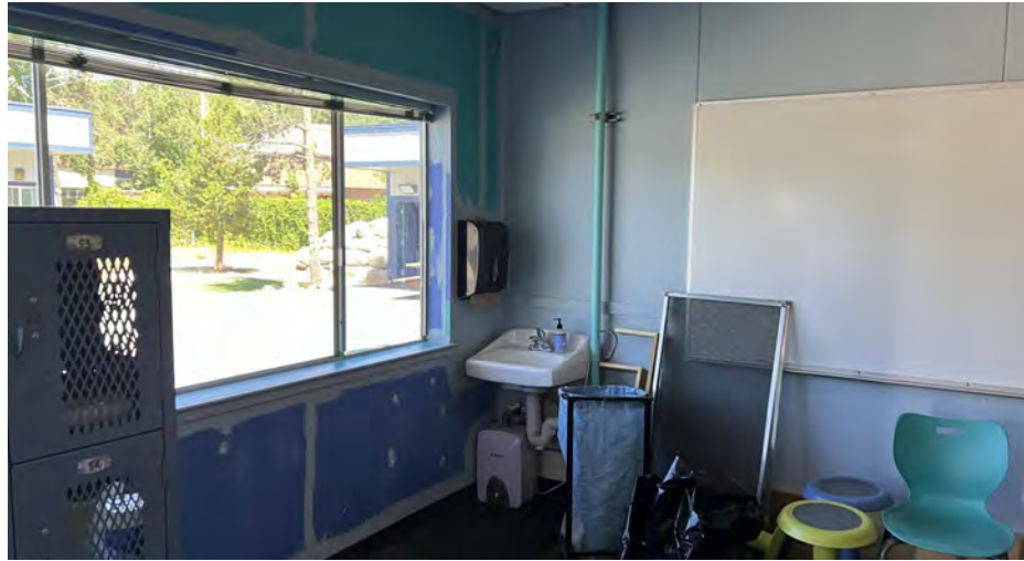
Interior paint and refresh at some areas
