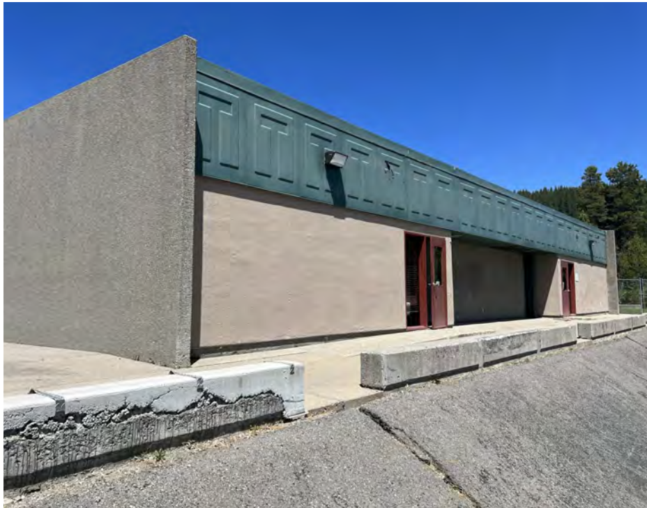
Hardscape and curb repaving
