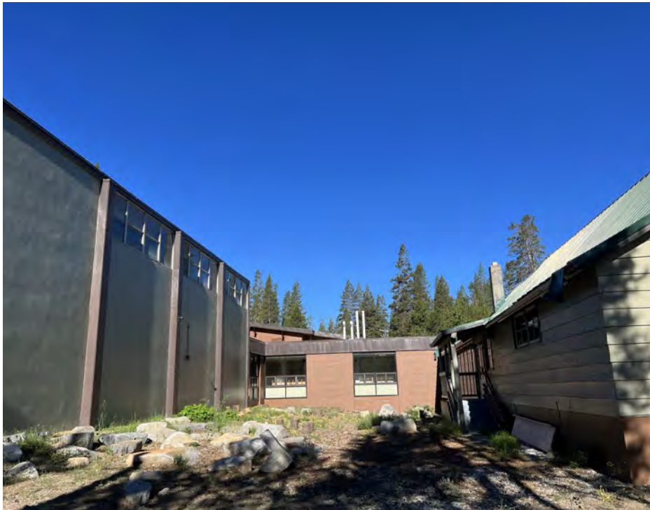
Roofing replacement and exterior renovation
