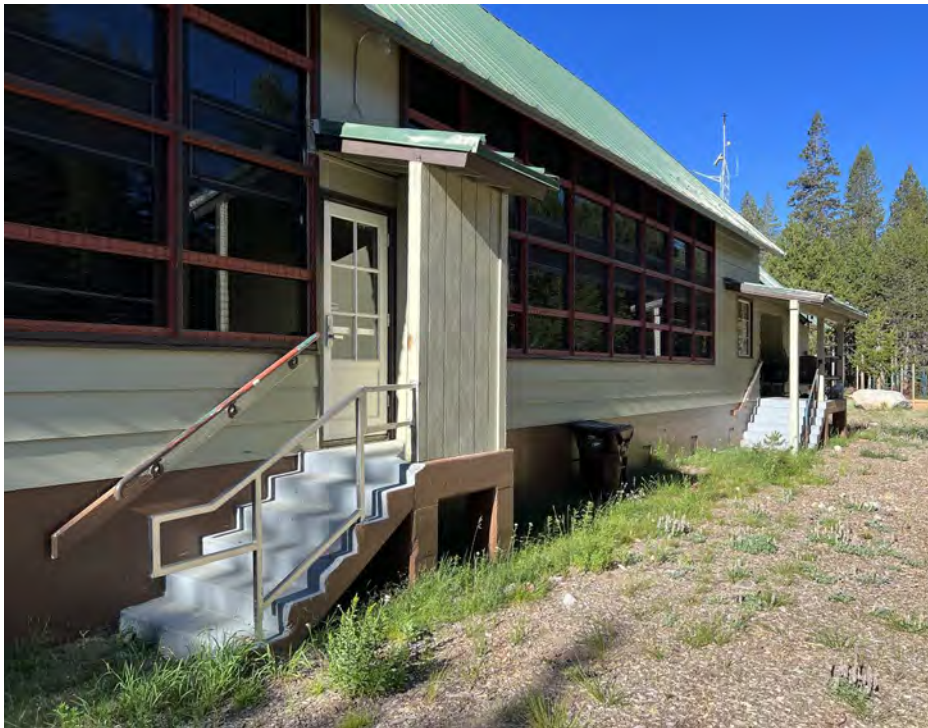
Emergency exit and site landscape upgrades
