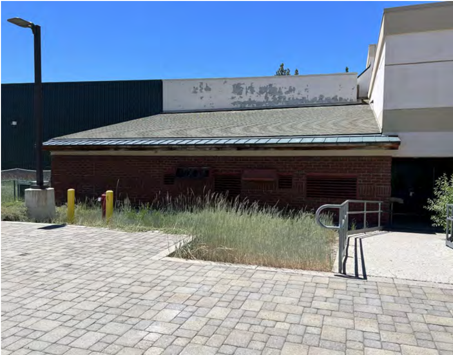
Exterior wall and paint replacement
