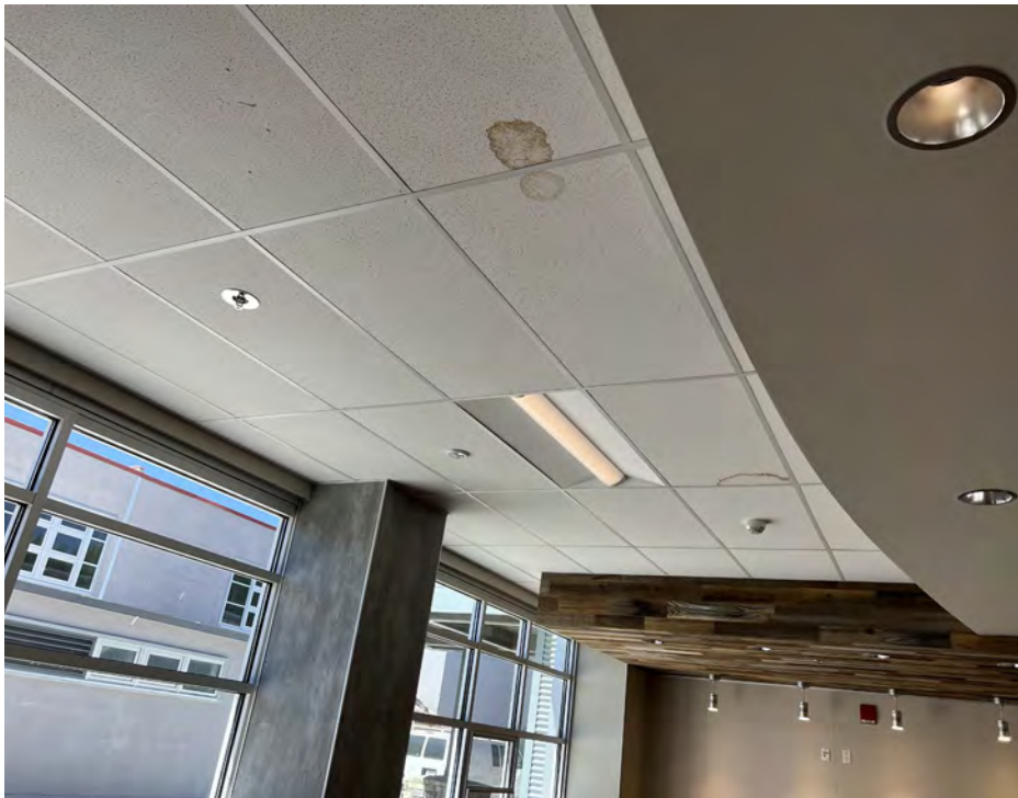
Acoustical ceiling tile replacement
