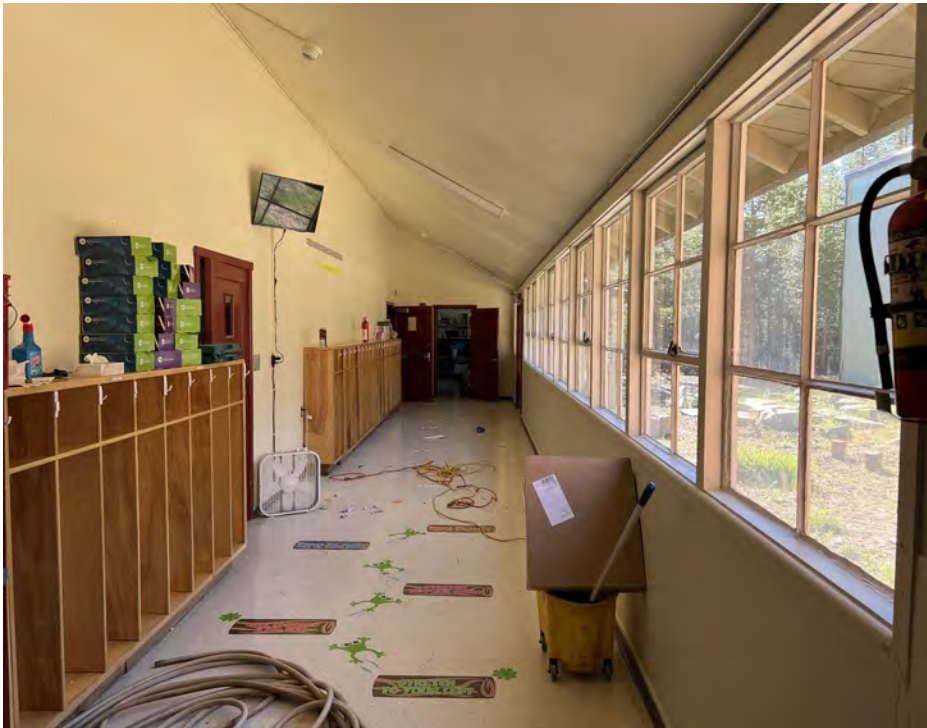
Interior finish upgrades and replacements
