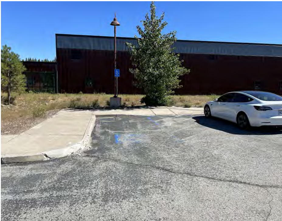
Curb Replacement and restriping
