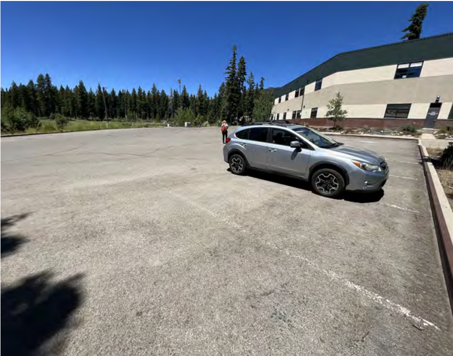
Parking lot asphalt upgrades
