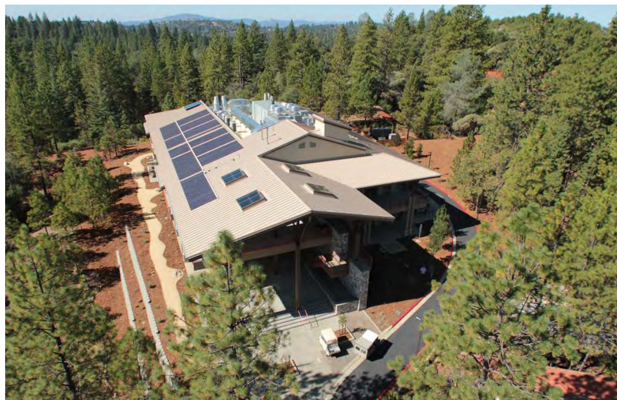
Rooftop Solar Photovoltaic Panels
