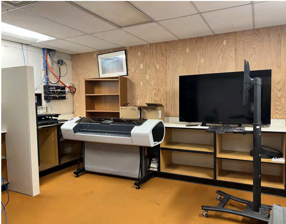
Interior finishes and casework modernizations
