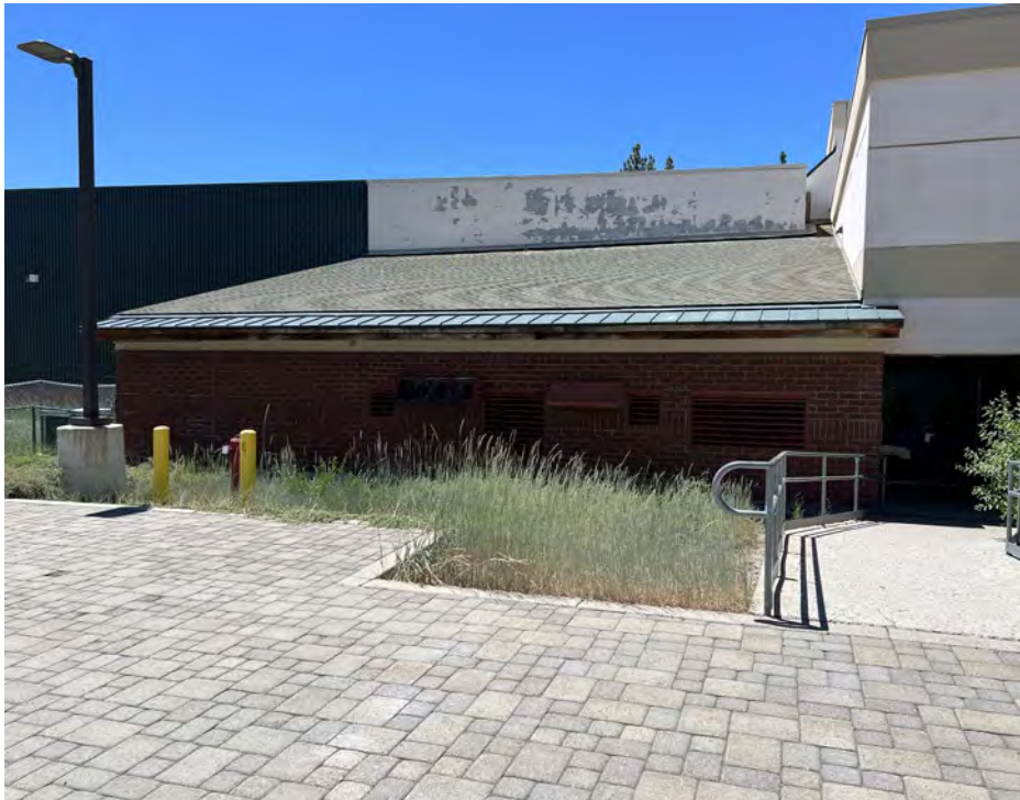
Exterior wall and paint upgrades
