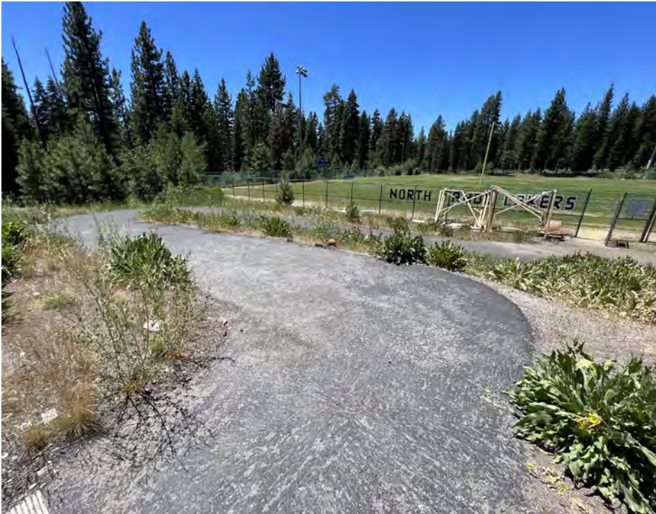
ADA path upgrades to the field
