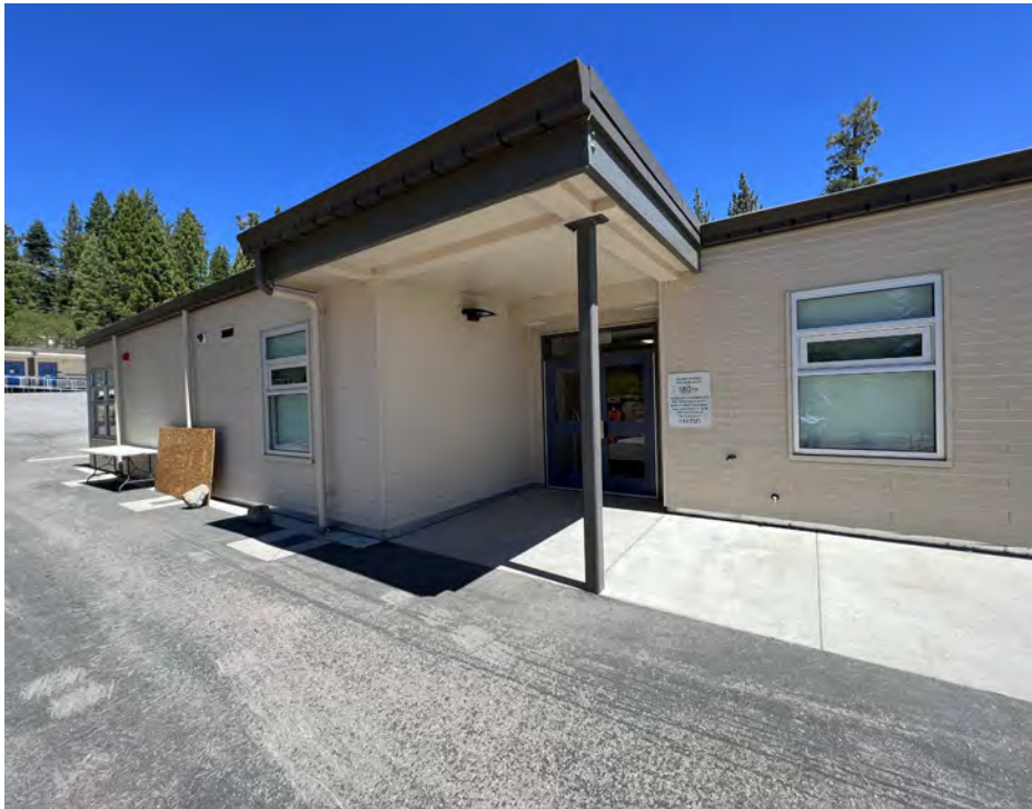
Roof, windows, and concrete upgrades
