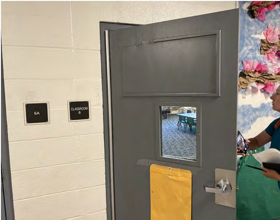
Classroom door and interior renovations
