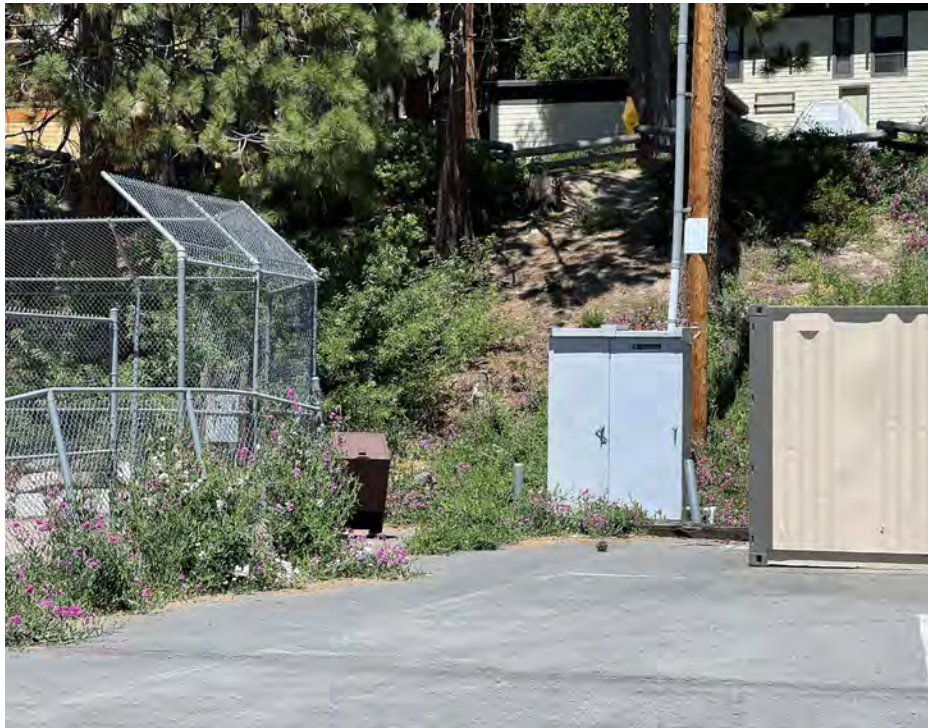
Perimeter fencing and gates needed
