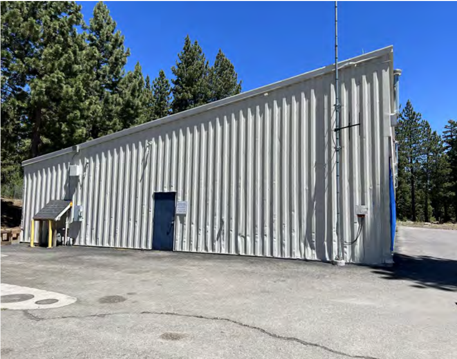
Exterior lighting and facade upgrades
