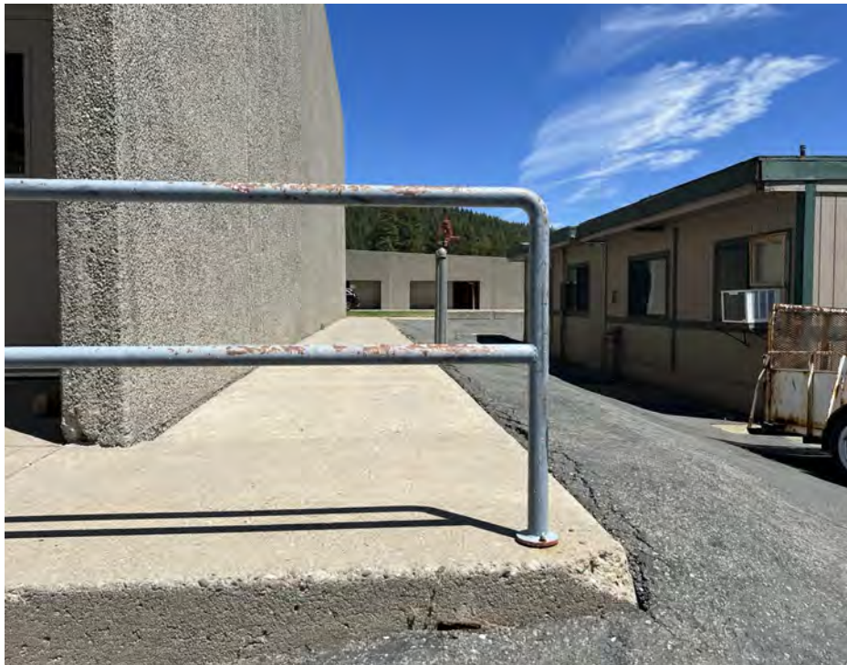
Curb, asphalt, and rusted handrail replacement
