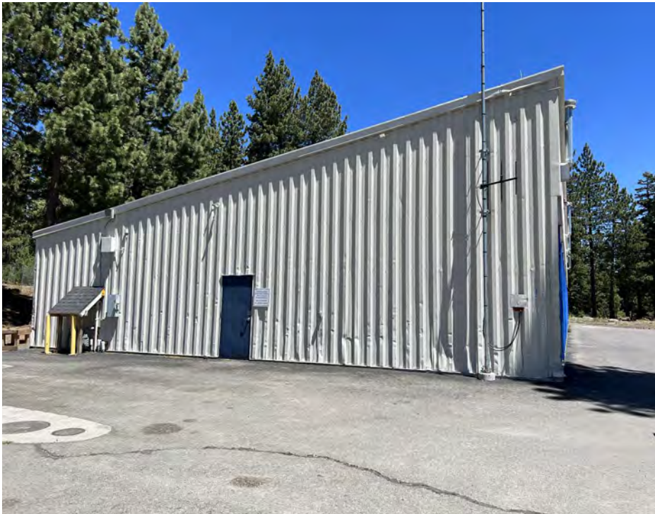
Exterior lighting and facade upgrades
