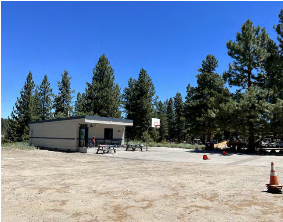
Landscape improvements and hardscape repavement
