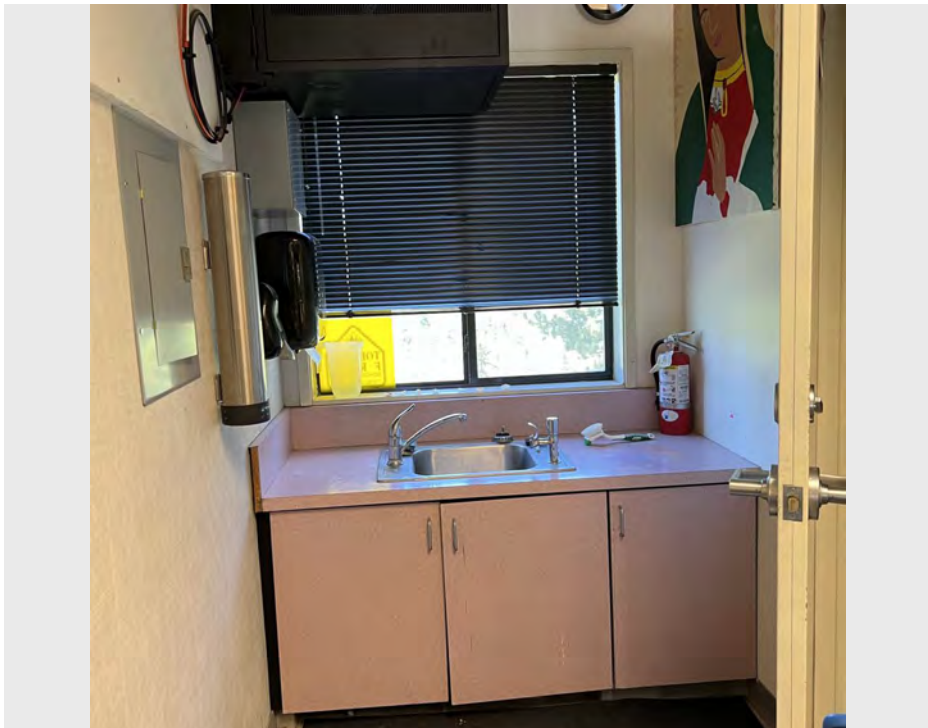
Interior finishes and casework upgrades
