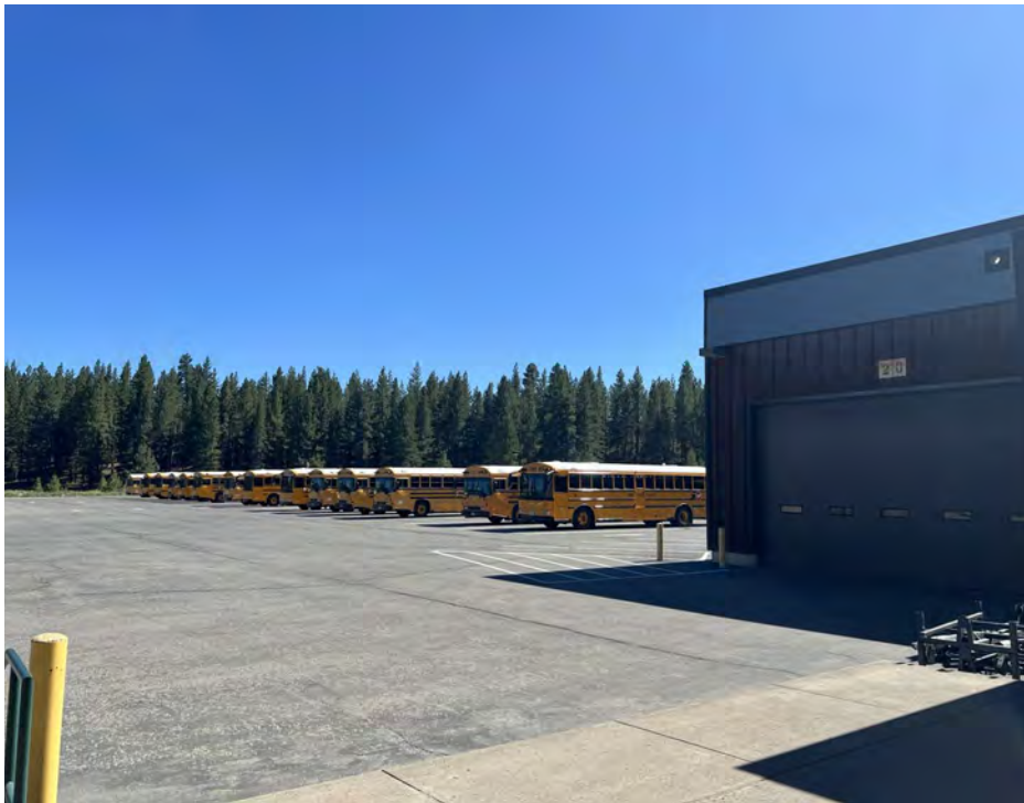
Loading dock and parking lot
