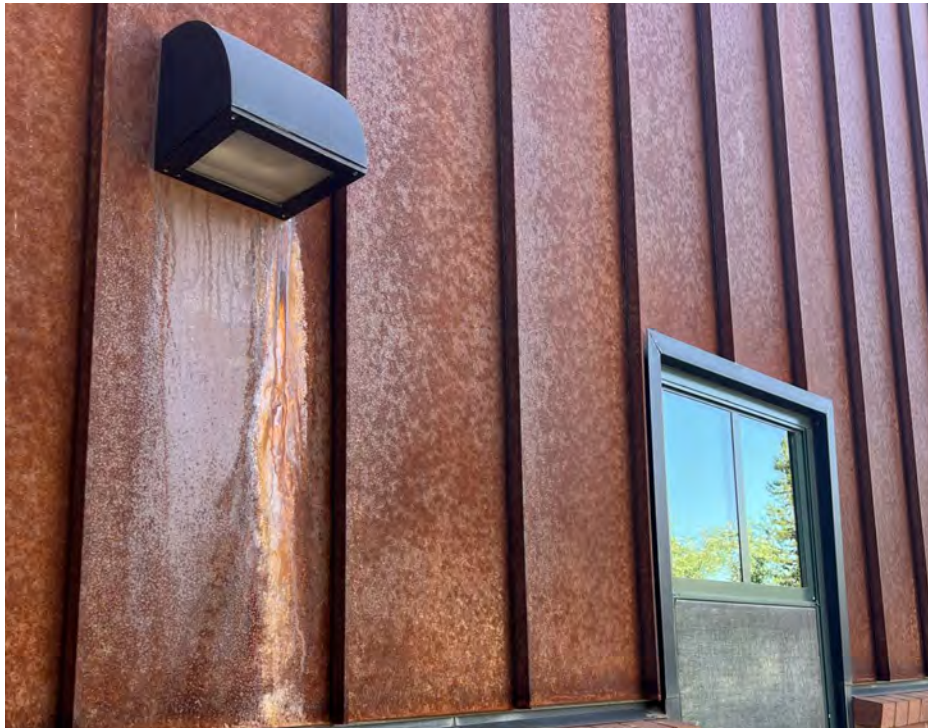
Exterior facade upgrades
