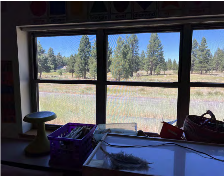
Snow removal access needed for windows
