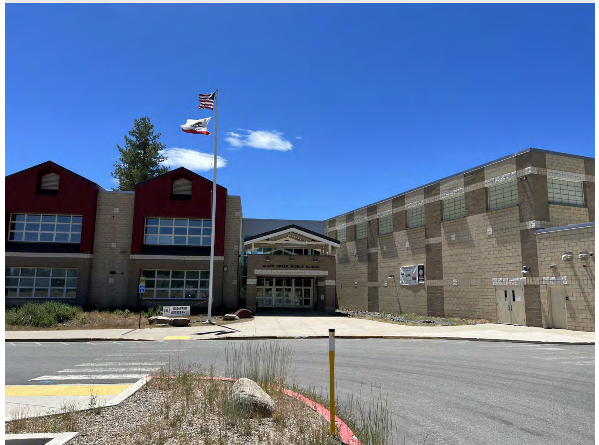
Entrance at Alder Creek Middle School
