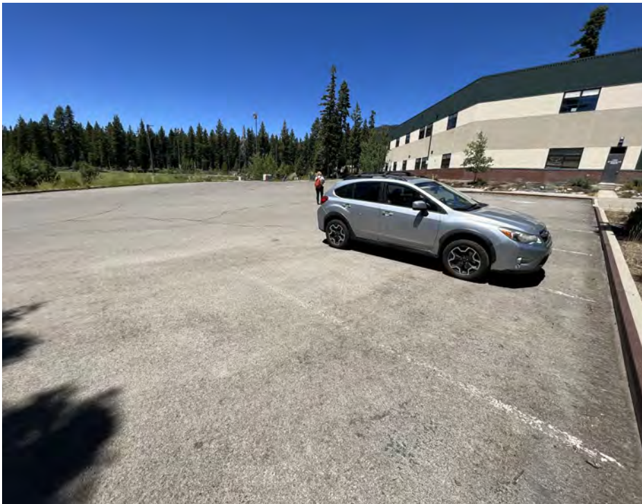
Parking lot asphalt upgrades
