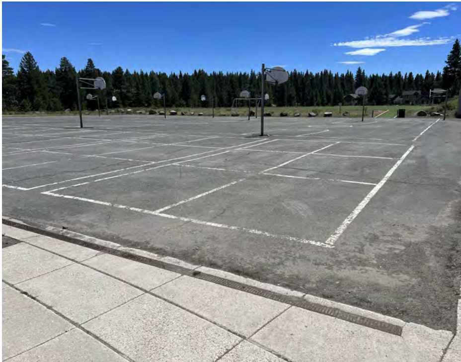
Hardscape courts and playground upgrades
