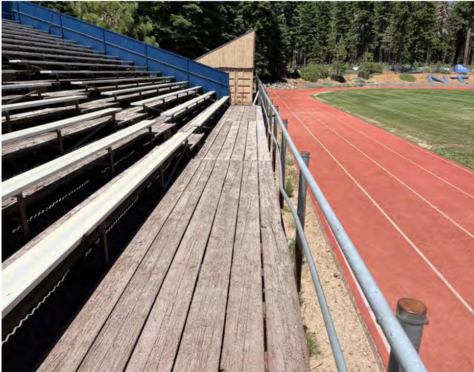
New stadium bleachers
