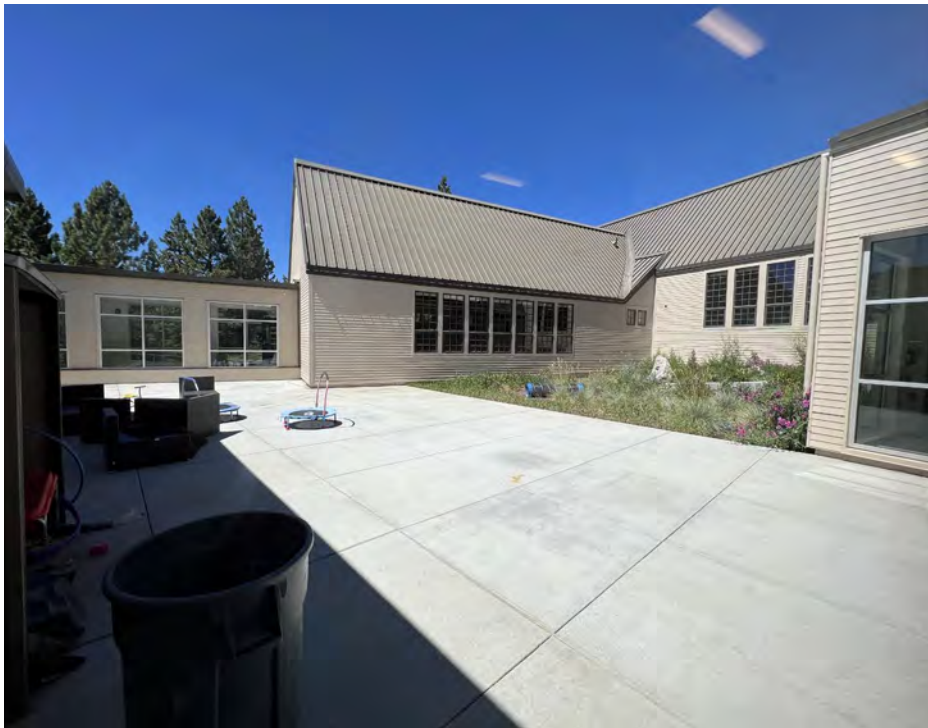
Upgrading outdoor spaces
