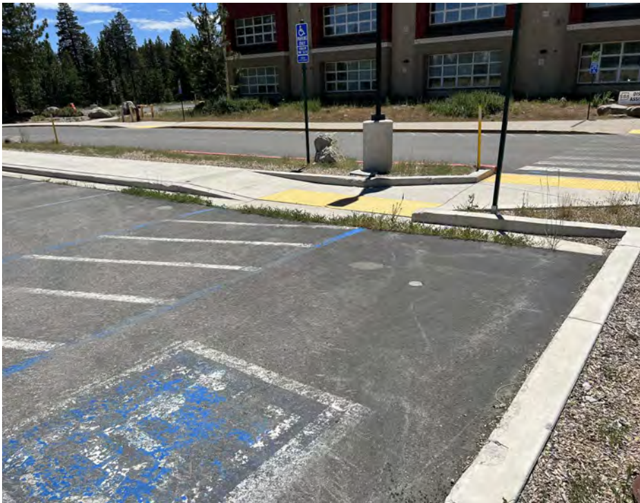
Asphalt in parkinglot and drop-off paving upgrades
