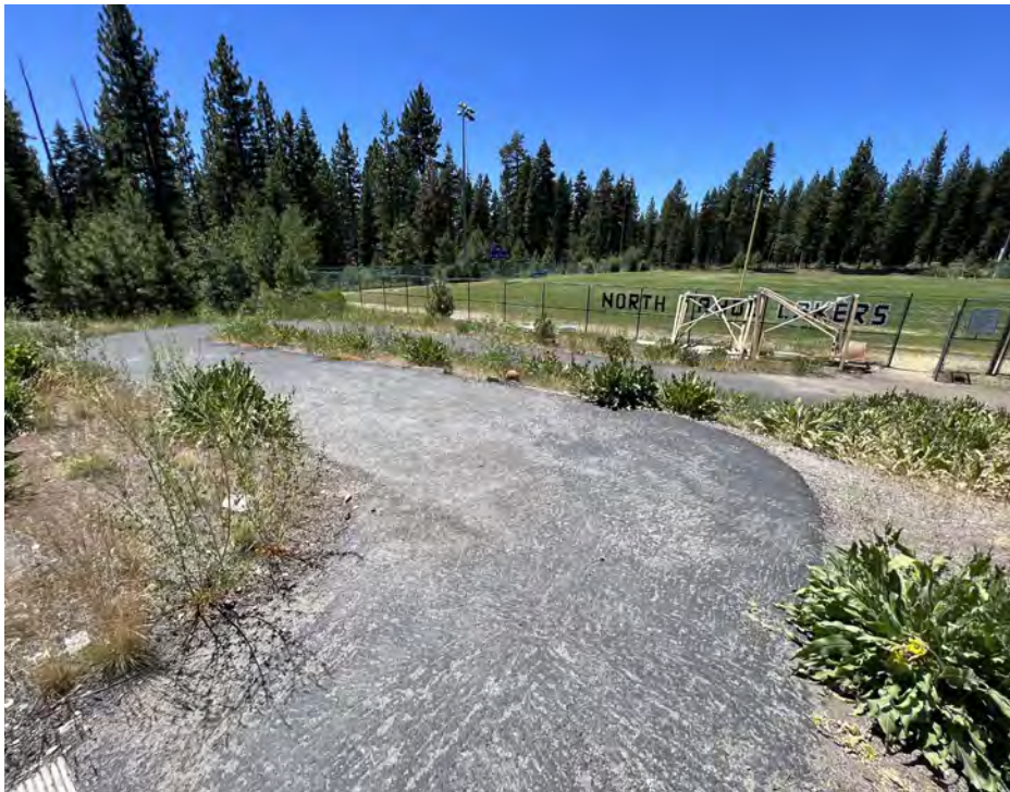
ADA path upgrades to the field
