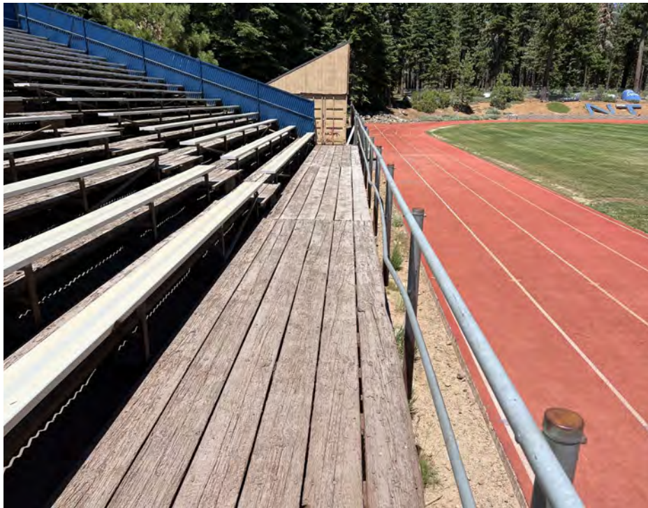
New stadium bleachers
